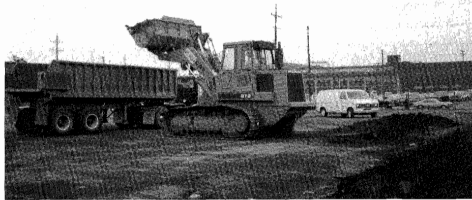
Ground was broken on July 10 for the $2.5 million Nail Department Shipping and Warehouse facility.
