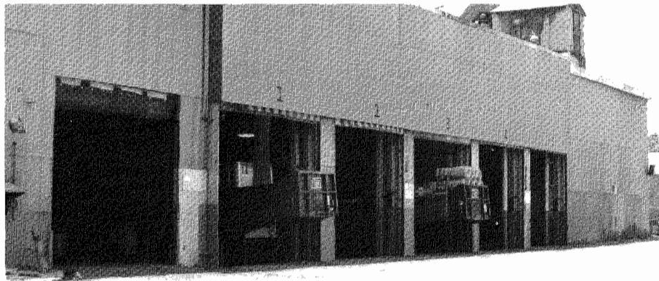
The H.O.P.E. Team has come up with several suggestions for reducing heat loss at Plant 4. Many of the solutions focus on the shipping doors.
