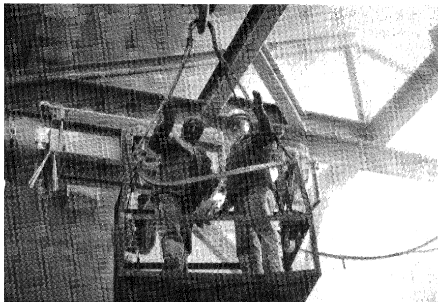
Maintenance workers who installed new ladle cars on the casters at NSW this winter had to brave sub-zero temperatures to get the job done, however, the team effort resulted in an installation target date being met.
