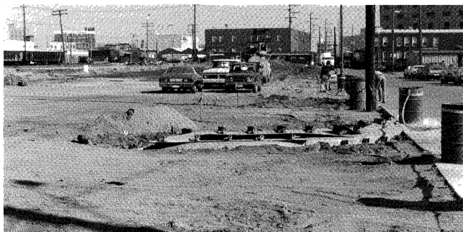
The parking lots near the print shop and office annex at NSW were recently expanded and paved. According to NSW officials, the final phase of the project will include striping the lot and adding lighting.
