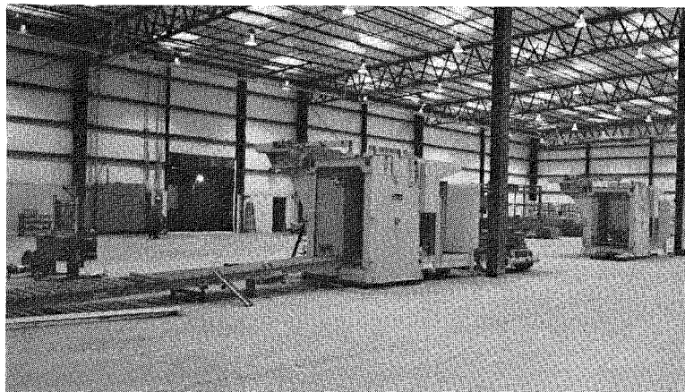
Shown are portions of the new palletizing machines at the new Nail Packing Facility.
