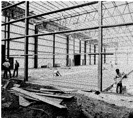
Workmen pour paving for the shipping dock at Northwestern's new Nail Packing Facility.
