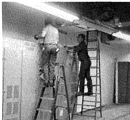
Workmen install electrical equipment in the computer room of the new ASEA speed control system at the 14-Inch Mill.
