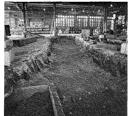
Excavation for the 120-foot coil conveyor which will carry compacted coils into the 12-Inch Mill and 46-Inch Mill bay for storage and shipping is shown above.
