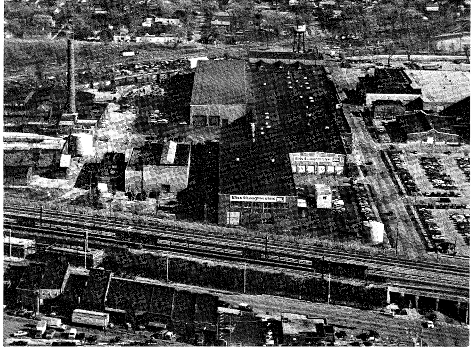
Shown is Bliss & Laughlin's Harvey facility which includes the biggest drawbench in the U.S. The 650,000 lb. draw bench has a capacity to make rounds from 3/4" to 6". Northwestern produces Hot Stock for Bliss & Laughlin's cold drawn bars.
