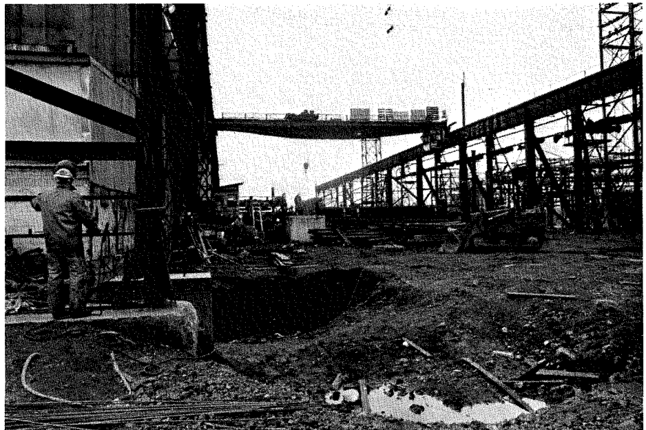
Construction is currently underway to install seven new concrete piers and eight new steel columns at the 12-Inch Mill Conditioning Yard.
