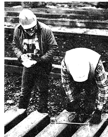
Sam Amasquita, Turn Foreman (right), and Gene Simmons, Stocker, are shown checking the size of the slab to make sure it's in section.
