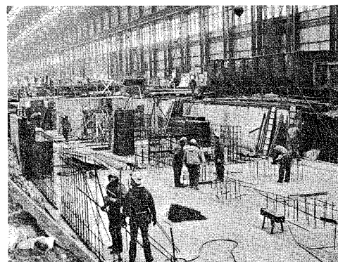
The construction never stopped inside the 14-Inch Mill where the workers were protected from winter's winds. At the left is a view of the in-line straightener roll-out line excavation. The center photo looks east at the new cooling bed roll-out tables. Work on this phase is nearing
